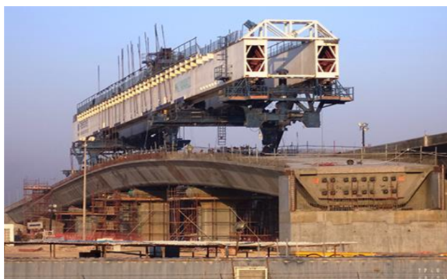
Figure 7: Precast Dammam Bridge (Freyssinet, 2022a).
