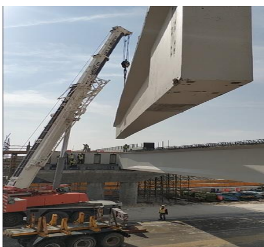
Figure 8: Rail Over Precast Bridge (Kanellopoulos, 2019).
